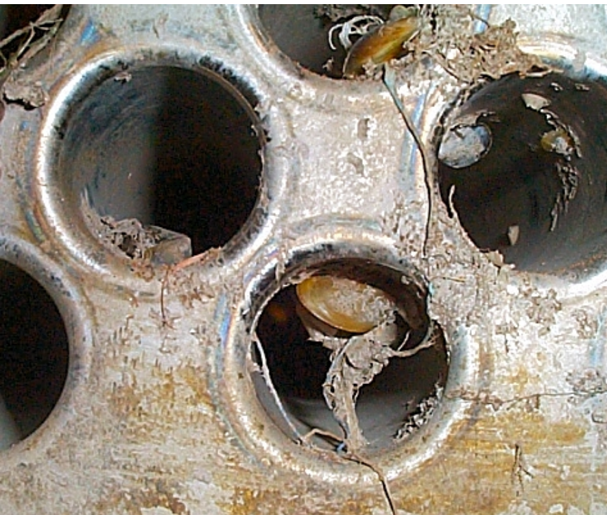
Mussels within the condenser tubes of a power station.
